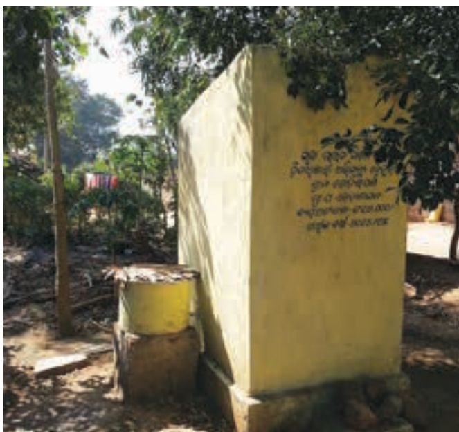
An elevated water tank connected to the tap, an innovation to ensure tapped water supply in Angul, Odisha
