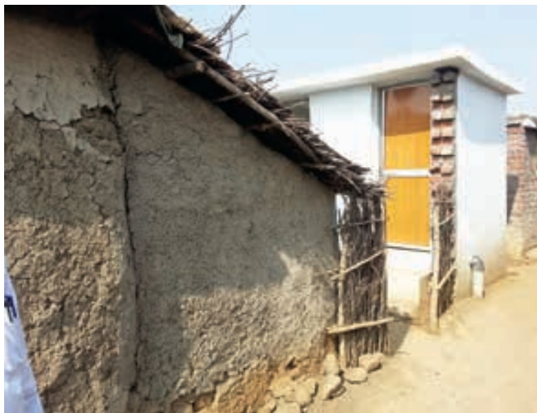
Public participation - The villager in Dhamangaon, who lives in a hut, has built a concrete toilet with the help of Rs. 12,000 from SBM funds
